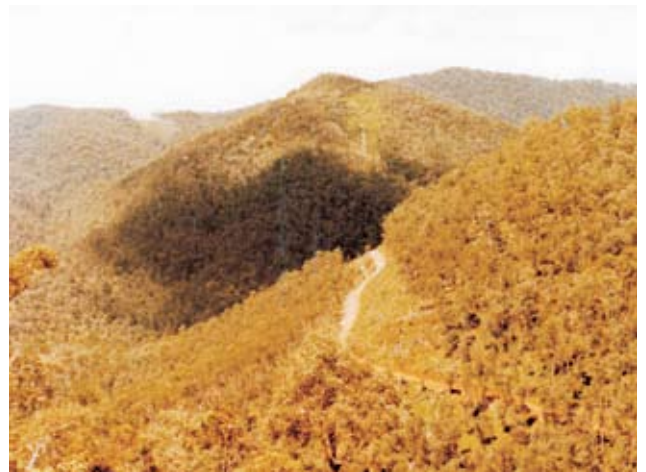
11 spans flown in Victorian Alps - Dartmouth to Mt Beauty Power Station
